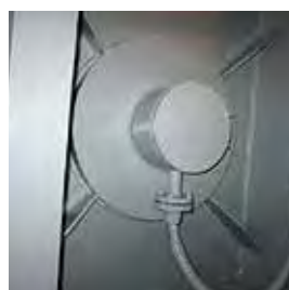
Anode internal view
